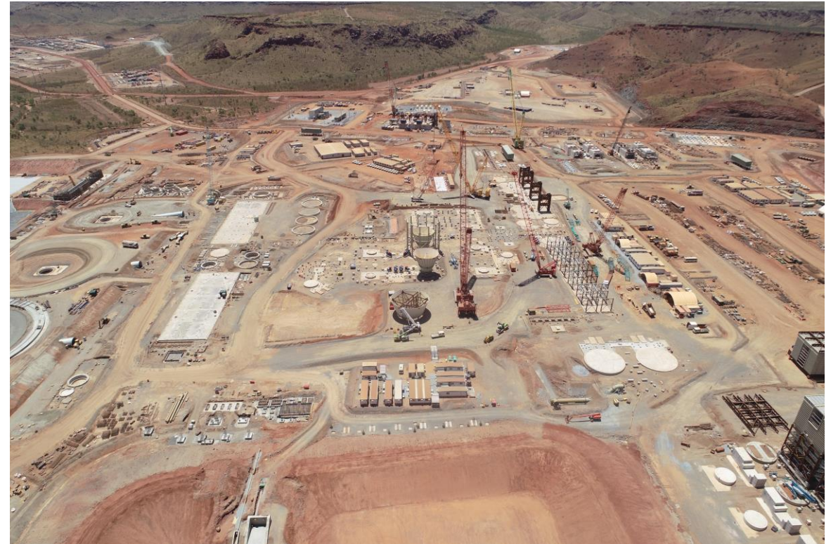
Construction of the ore processing facility
