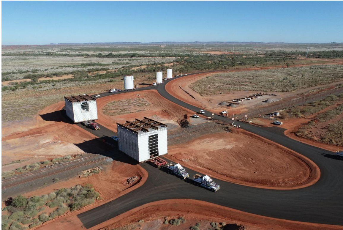
Delivery of large modules to Iron Bridge
